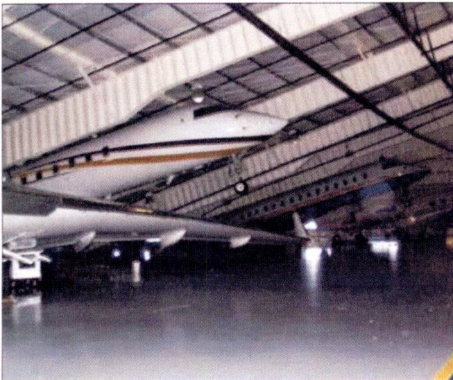
The collapsed roof at Dulles Jet Center in Washington, D.C. Insurance companies faced a bill for millions of dollars in damages after a massive snowstorm hit the U.S. East Coast in February 2010.
